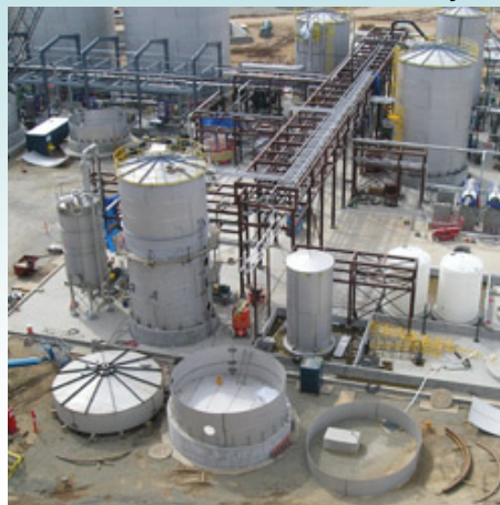
Pacific Ethanol Madera Refinery
