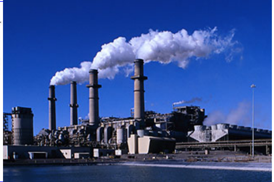
CCS power plant
