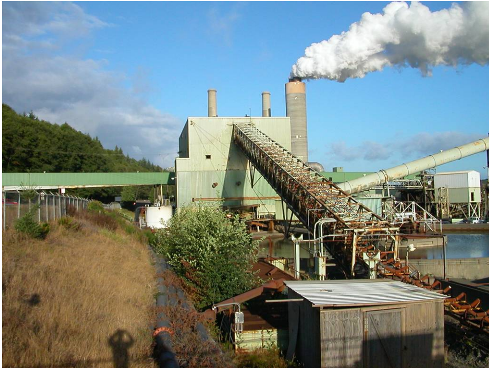
Centralia Generating Station
