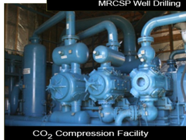
CO 2 Compression Facility
