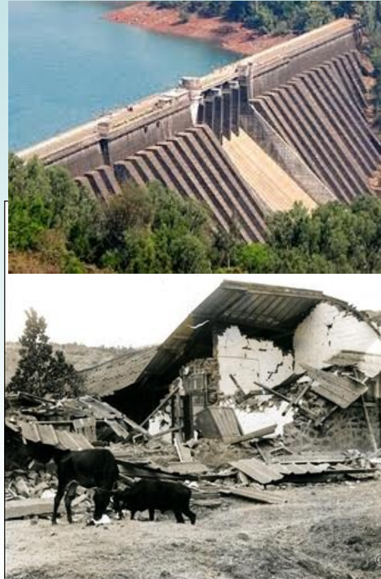
Koyana reservoir dam, India, (above) and damage from 1967 M6.5 earthquake (below) ( www.indianetzone.com and www.timescontent.com )
