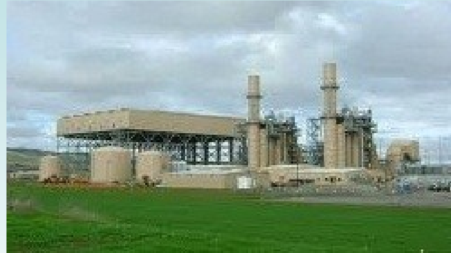
PG&E's Colusa Generating Station (in-service December 2010)
